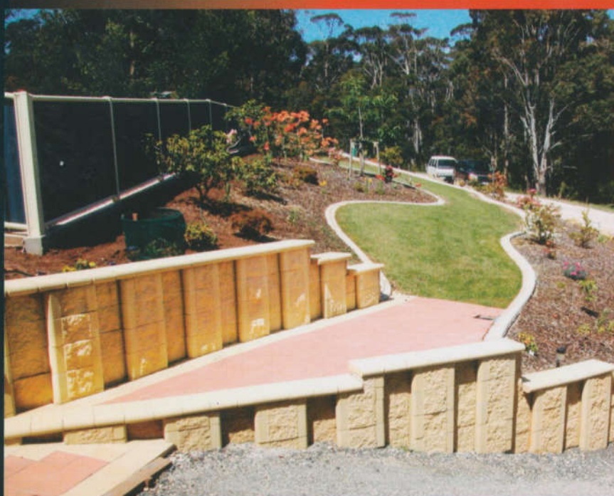
Spectacular retaining wall for your driveway
