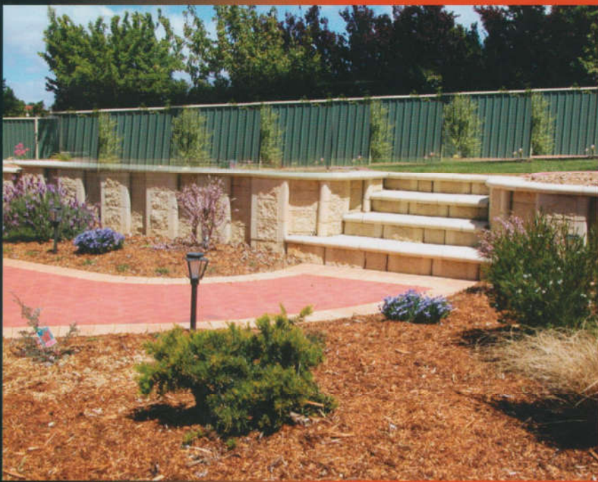
Retaining wall with a step insert
