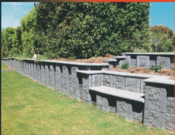
Flowing retainer incorporating seat
